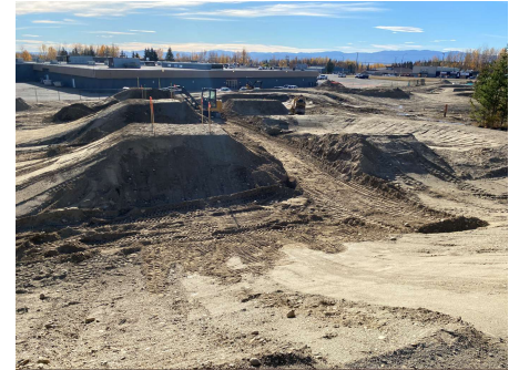
Flow Track under construction
